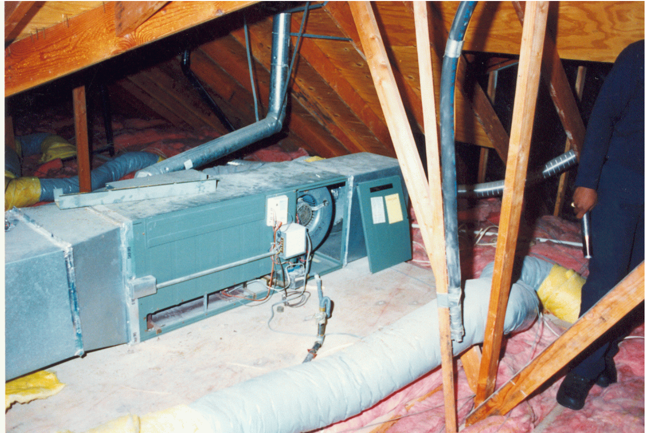
Photo One: Typical installation method for H-Series furnace.
