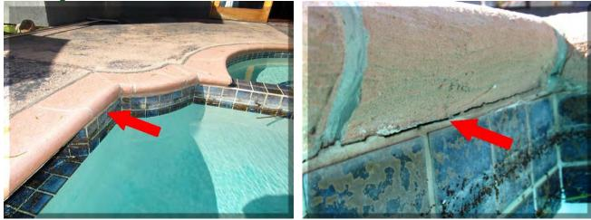
4. The mastic sealant between the deck and coping is deteriorated/cracked. Water entry will occur causing settlement or heaving of the pool deck.
