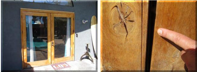
2. Moisture damage was noted at the bottom of the garage service door. Refer to the pest control report.
