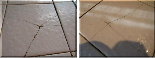
2. The countertop grouting is deteriorated. Water penetration will occur.
