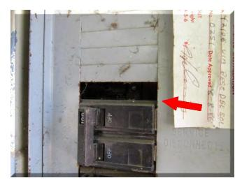
2. The circuit breakers in the electrical service panel are not identified. Unable to determine which circuit each breaker controls. Safety hazard.
