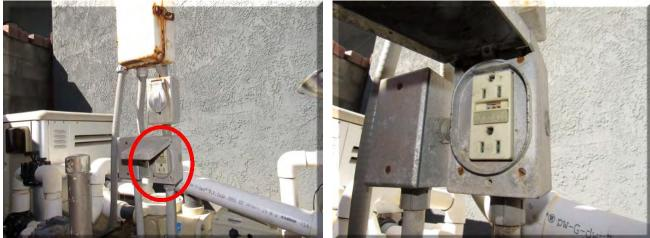
10. Missing components were noted at the pool/spa bypass valve handle. The valve is leaking.
