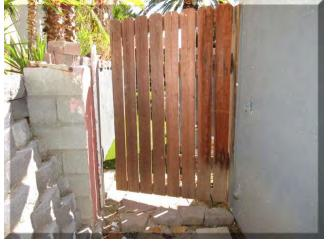
13. The opening under the pool-accessible gate is excessive. The maximum opening permitted is 2" to soil and 4" to hardscaping. Safety/drowning hazard.
