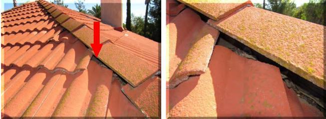
3. Water staining was noted at the roof eaves at the rear right corner of the home. Evidence of roof leakage at the rake edge. Further evaluation is advised.
