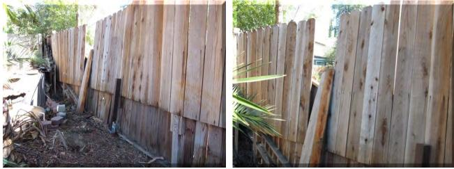
2. The gates at each side of the home have loose, missing or damaged components and do not function properly.
