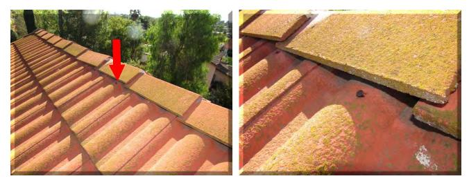
2. Numerous slipped tiles were noted at the hip ridges. Water intrusion will occur.
