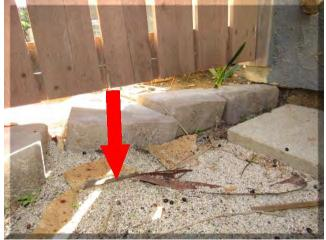
14. There is a climbable retaining wall adjacent to the exterior of the pool-accessible gate. The pool safety barrier can be breached. Drowning hazard. Correction is advised.
