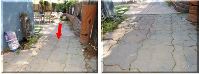
3. Several of the drain covers at the left side of the home are missing. The drains are clogged with debris. The drain near the front right corner of the home is also clogged with debris. Ponding water and excessive moisture conditions may occur at these locations. Although testing of outside area drains is beyond the scope of this inspection, the client is advised to consult a qualified licensed drainage contractor for further evaluation and testing.
