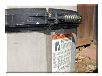
7. Manufacturers of band clamp filters, like the one at this site, require that the location of any switch that can activate a pump that sends water to a filter is installed at least five feet from the filter. This insures that the operator is a safe distance from the filter when the pump is activated. Exploding filter injuries are very serious and happen frequently despite low public awareness. Relocation of either the filter or control switches is advised.
